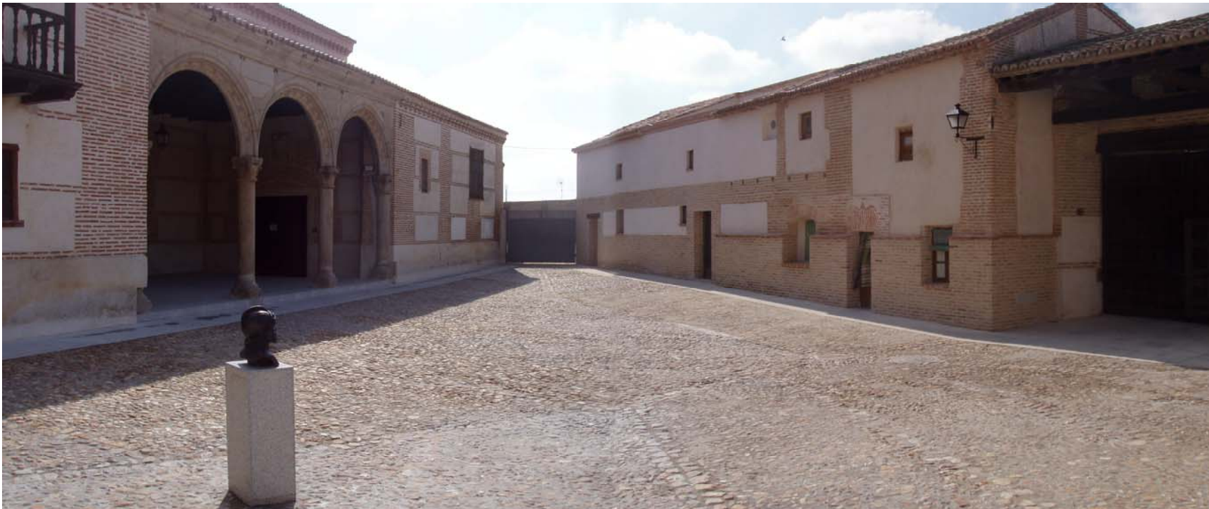
Courtyard to Monastery after restoration. General view.
