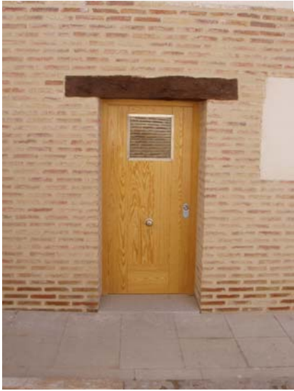
Entrance to multifunctional centre from monastery courtyard.
