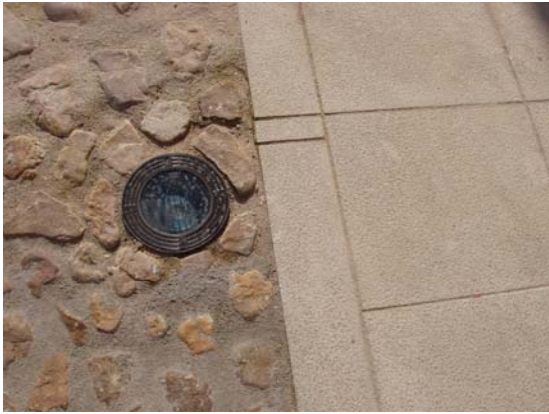
Lighting detail in entrance courtyard.
